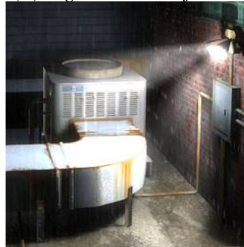
(c) Rooftop light cones
