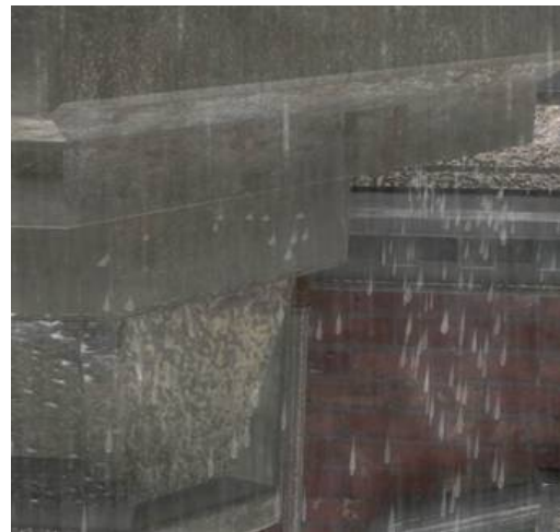
(b) Raindrops falling off the rooftop ledge
